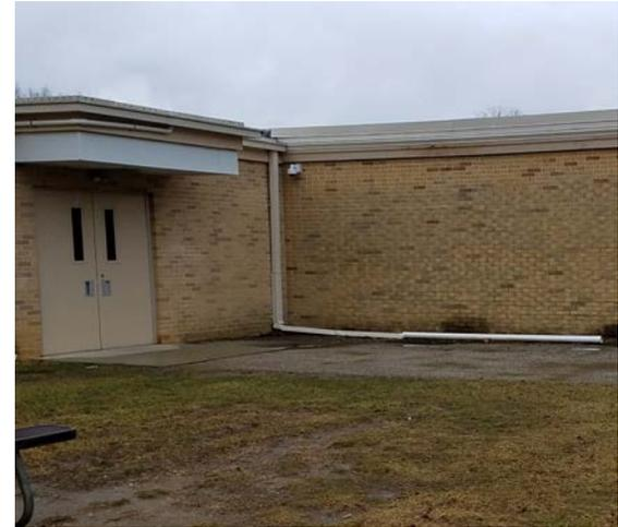
Rain gardens can be installed on both sides of the entrance to capture stormwater runoff from the rooftop. Pervious pavement can be installed in the parking spaces along the edge of the parking lot to capture additional stormwater runoff. A preliminary soil assessment suggests that more soil testing would be required before determining the soil's suitability for green infrastructure.
