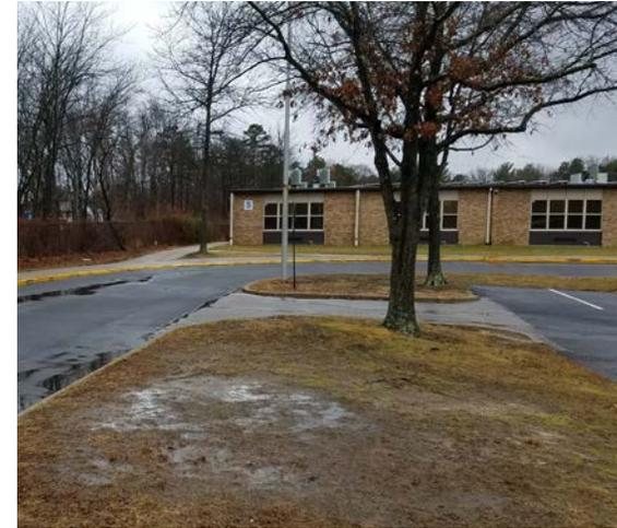
Rain gardens can be installed on both sides of the entrance to capture stormwater runoff from the rooftop. Pervious pavement can be installed in the parking spaces along with a bioretention system at the northeast end of the parking lot. This will hopefully also alleviate large areas of ponding occurring in that area. A preliminary soil assessment suggests that more soil testing would be required before determining the soil's suitability for green infrastructure.
