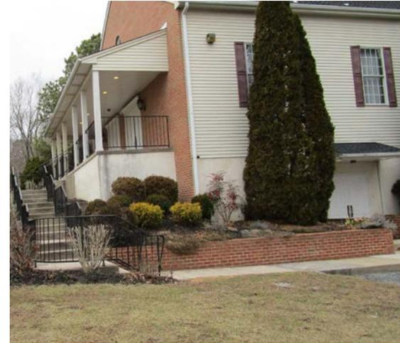
A rain garden can be placed near the northwest corner of the building to capture, treat, and infiltrate runoff from the rooftop. Pervious pavement can be installed in parking spaces on the site to capture runoff from the parking lot and rooftop. A preliminary soil assessment suggests that the soils have suitable drainage characteristics for green infrastructure.
